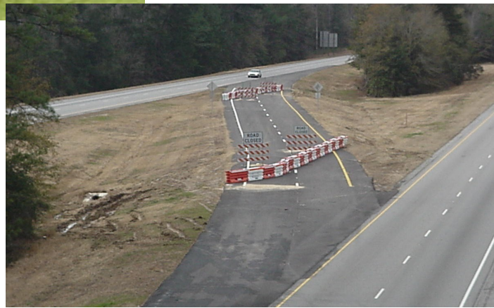
FIGURE 7. The first I-65 crossover for contraflow, near Mobile, Alabama. (Photo: ALDOT)
