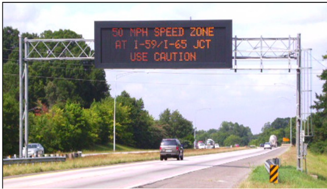
FIGURE 9. Bridge-type overhead VMS support structure
