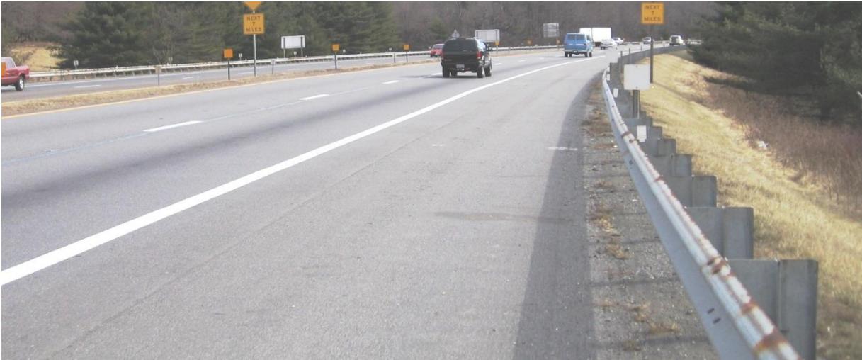
Figure 23. Photograph. An example of roadside barriers at the edges of paved shoulders.
